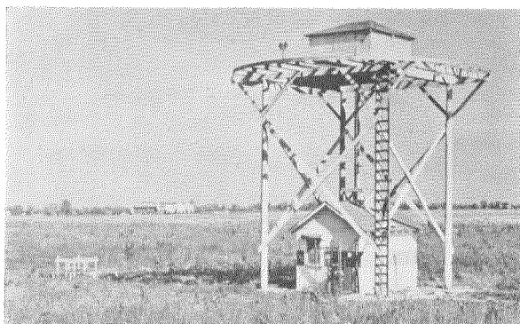
Fig. 16—Two-course radio range with sector identification and simultaneous voice, showing transmitter house, counterpoise structure, antenna house, and 125.020-megacycle marker.
